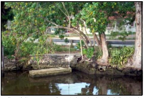
Figure A5: Limestone is a naturally occurring feature along the river banks. Here it is used to build a retaining wall along a portion of the River.
