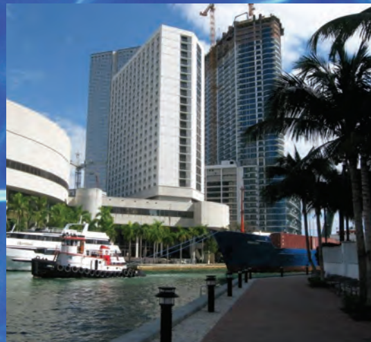
BELOW: Miami River Greenway along the Lower River south bank with vessel under tow.
