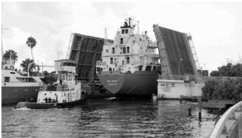
THE FIFTH STREET BRIDGE – only 74 feet wide on a 150-foot channel – is the most restrictive point on the river, a hazard for navigation, and a common site for collisions. Freighters have struck the bridge 12 times in 10 years, twice knocking out service for eight months. We urge the Florida Department of Transportation to replace this unsafe bridge promptly. Three of the river's 15 bridges are more than 70 years old and in urgent need of replacement. The commission recommends aggressive study of tunnels as an alternative to bridges.
